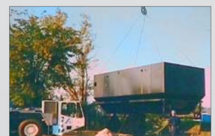
System anchored to Foundation Slab. Ancillary equipment, blowers & controls are placed
