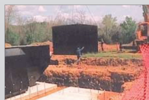
Tertiary Filter System is set into position
