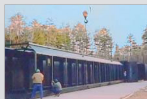
Sections are re-assembled and made watertight. Additional sections set into position
